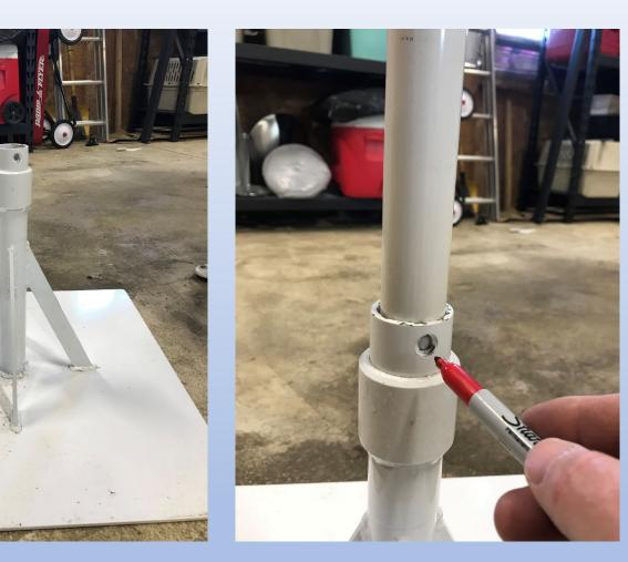
Install lower post into base or in-ground mount
